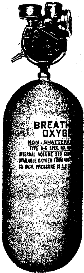
Figure 12. Type A-1 Portable Oxygen Unit, Diluter Demand.
