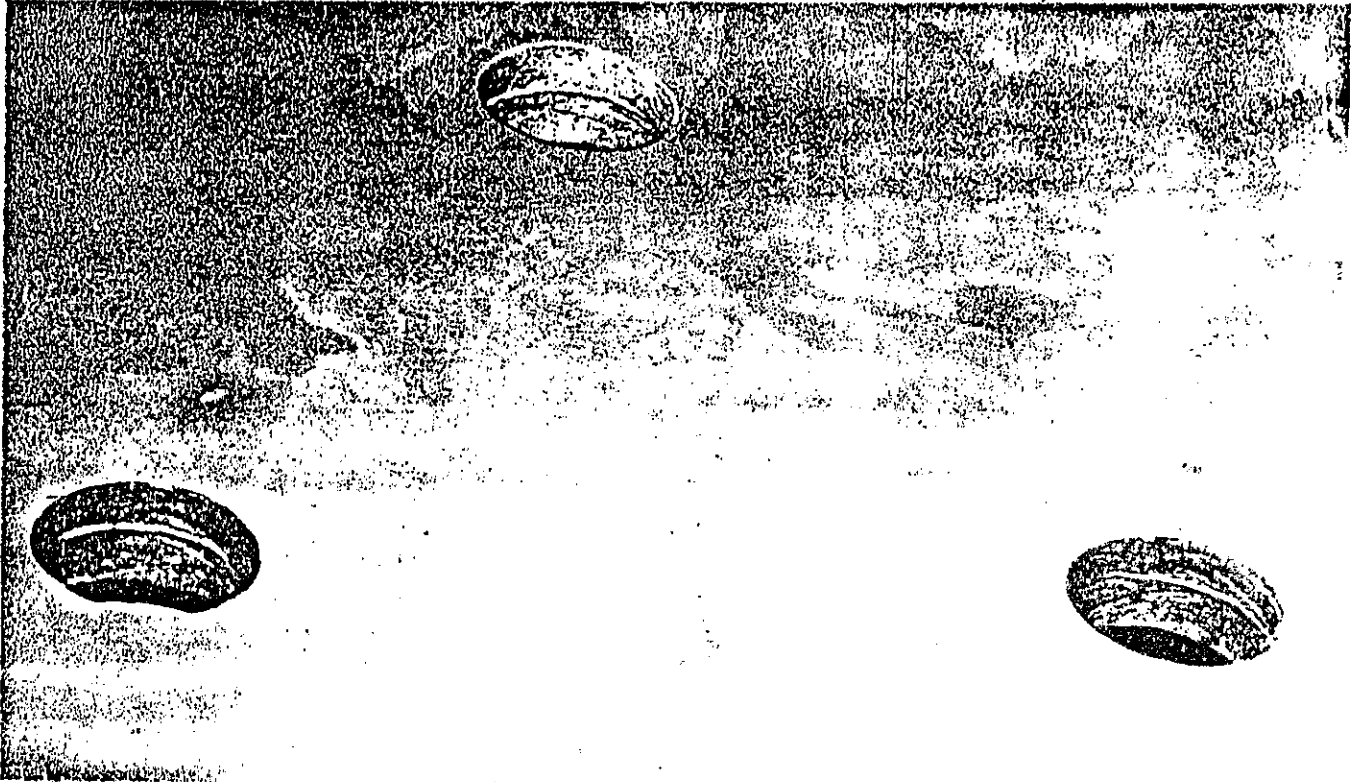
Fig. 10. Seams in Boiler Plate
